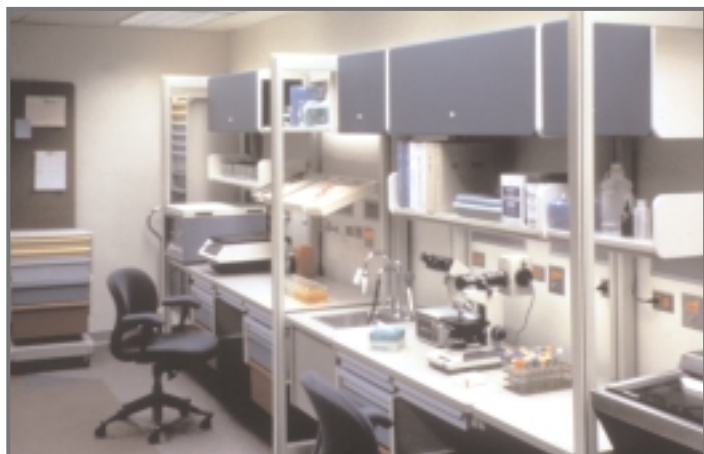
Coordination with wall mounted electrical and mechanical equipment is necessary to avoid conflicts.
